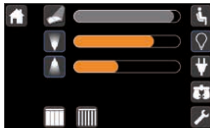
Dimming of room light and reading light by swiping the touch screen. Control of open and close of the curtains.
